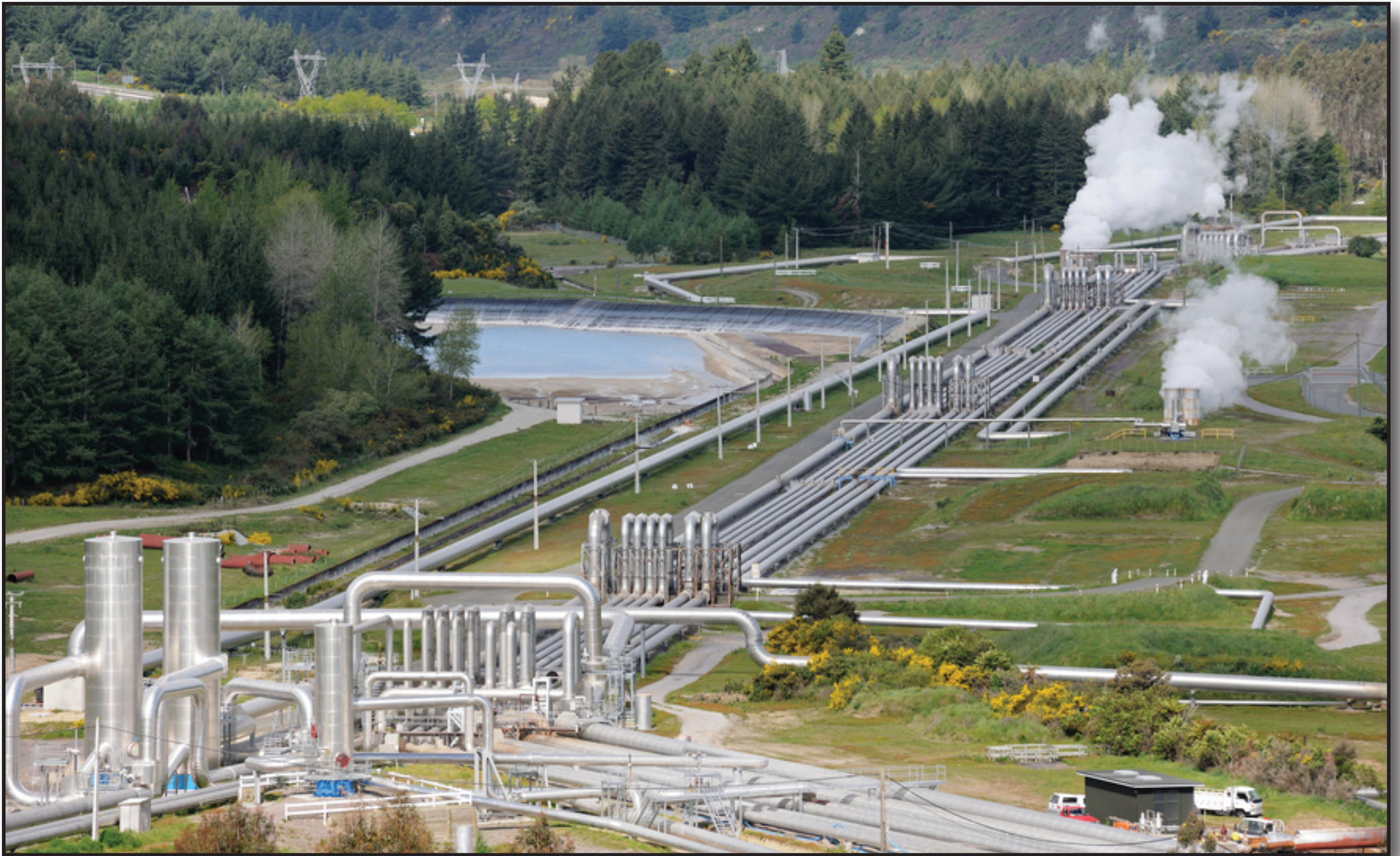
Wairakei Power Station in New Zealand's north island.
