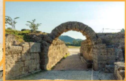
Crypt (arched way to the stadium)
